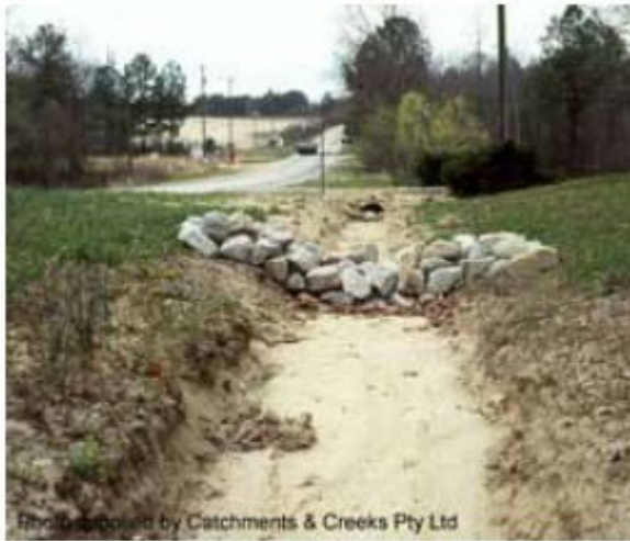
Rock check dam
